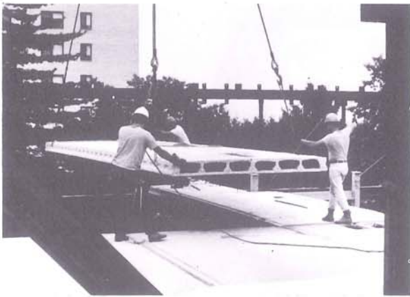
Large sections of precast, prestressed concrete planking for walls, floors and roofs of schools, warehouses, motels and shopping malls are a product of MCS.
