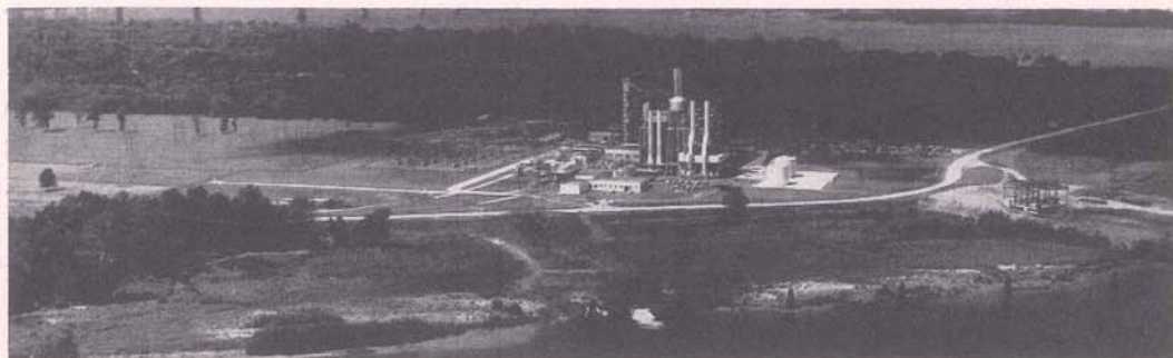
Abundant good water from the Mississippi River is one of the chief reasons Louisiana Power and Light Company located this Nine Mile Point steam-electric Generating Station near Westwego in Jefferson Parish. It circulates 300 million gallons of river water per day through its cooling system. The land tip of Nine Mile Point is not shown in this photograph, but both bodies of water are the Mississippi. The bridge is the Huey P. Long train and vehicular bridge opened to traffic in 1935.
