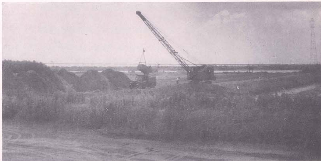
Loading river sand that was hydraulically dredged from the Mississippi at Jahncke Service's East Bank pit up river from the Huey P. Long Bridge seen in the background. Each year from the sand pits on both sides of the river about 3,000,000 cubic yards of sand is trucked to industrial or home building sites in Jefferson Parish. Thousands of building sites in the parish have been raised a foot or more with the top soil from the thirty-one states that drain into the Mississippi.
