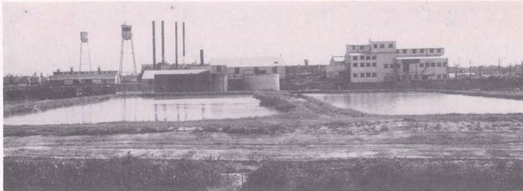
The settling basins at the Celotex plant (background) in Marrero where the raw river water is held for three hours to allow silt to settle. These basins can hold 4,200,000 gallons of water. They are a lush habitat for the famous Mississippi River catfish which are pumped in as babies and grow into king size specimens. Big strings of "cats" are taken from the basins each year when they are drained to be cleaned.
