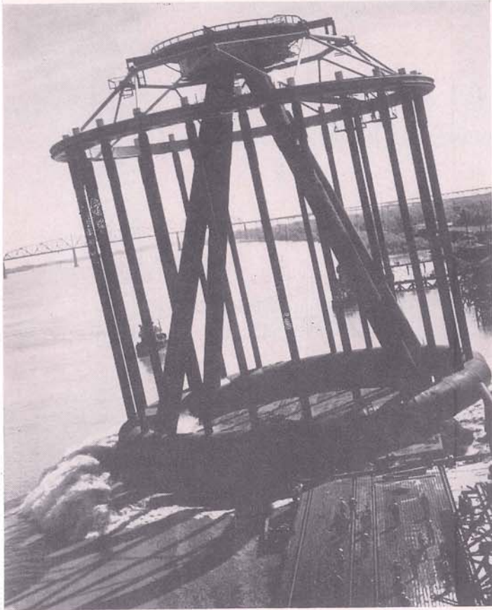
A massive offshore loading platform is launched at Avondale Shipyard's main yard. Its destination the Coast of Libya in North Africa. Notice the comparison in size between the men in the foreground and this mighty platform.
