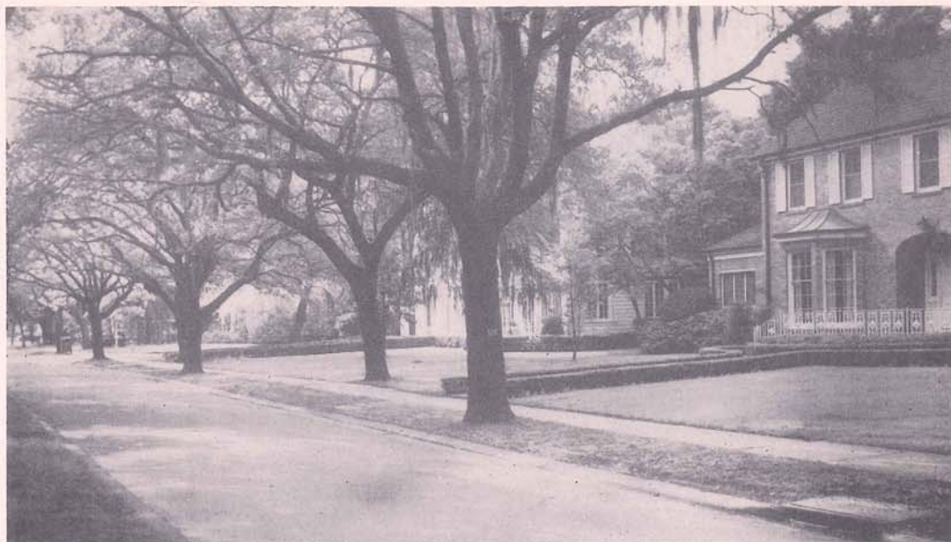
As shown, the asphalt paving of Northline in Metairie, with 8" vertical curb around neutral ground and roll over curb on lower side, was completed by the Department of Roads and Bridges in November of 1961.
