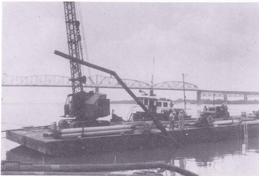
Louisiana Gas Service Company of Harvey lowering four 10 inch pipelines under the Mississippi River at Nine Mile Point carrying natural gas between the East and West Banks of Jefferson Parish.
