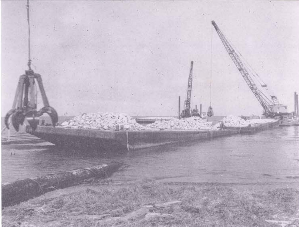
The Rock Jetty at the east end of Grand Isle under construction by the Louisiana Department of Public Works for the protection and stabilization of the gulfward beach of the island. It will cost $124,336 and will be a jetty of heavy stone resting on a timber mattress extending approximately 800 feet into Barataria Pass. It will require 1524 tons of ballast stone, 5807 tons of jetty stone and 60,300 square feet of timber mattress. When completed it will act as a barrier to eastward drift and loss of material from the shore of Grand Isle. Before it was started 125 feet of beach front had been lost in this area.
