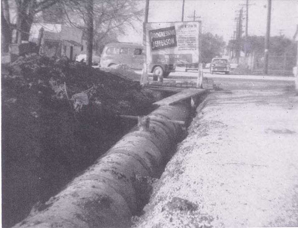
A close up of a current drainage project of the Jefferson Parish Sanitation Department—an $8,000 job to eliminate the flooding condition along the highway known as the Marrero-Westwego Highway in front of the Celotex Corporation plant in Marrero.
