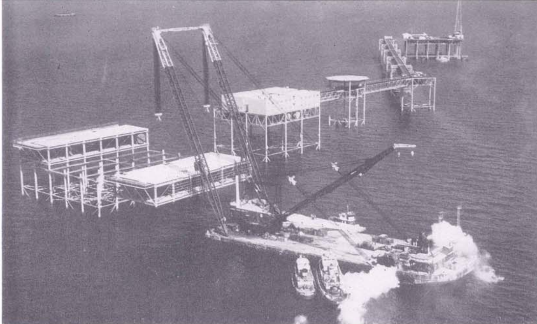
The J. Ray McDermott and Company special rig for the 800 ton Lift Derricks used to place in position the installations of the Freeport Sulphur Mine platform 75 feet above the Gulf and 7 miles off the shore of Grand Isle. This is the heaviest floating lifting equipment in the world. It is shown lifting a deck section of 645 tons. The boom on the big derrick is 250 feet long. The little revolving derrick has a 250 ton lifting capacity. J. Ray McDermott built, delivered and installed with its special derricks this entire Freeport operation which will be 75% complete by January, 1960.
