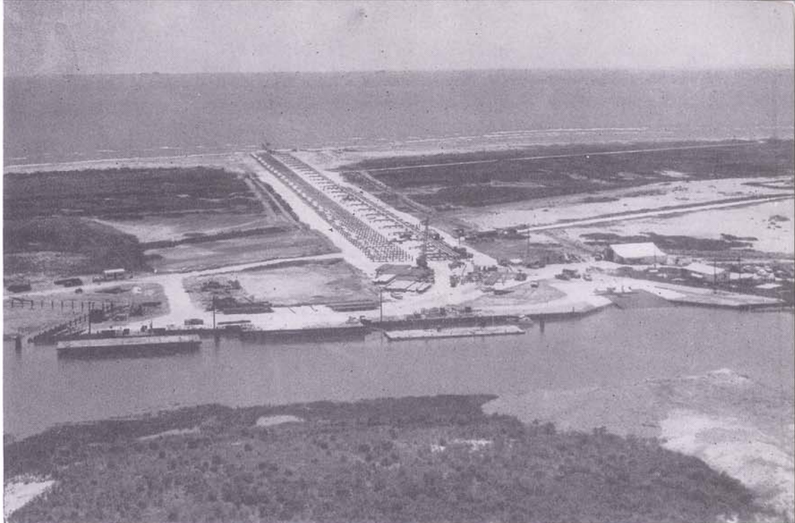
Aerial view of the pipeline being connected on the east end of Grand Isle which will pipe the molten sulphur to the Grand Isle base from the Freeport Sulphur Mine 7 miles offshore. Basically the pipeline will transfer the molten sulphur into Freeport's unique "thermos bottle barges" at the Grand Isle base. It is then transported 25 miles to Port Sulphur where it will be pumped ashore and allowed to solidify. The pipeline is a six inch line inside a 7 1/2 inch line and the space between carries water heated to 320° F. Covering this water jacket is a thermal insulation 2 1/2" thick. All this is encased in a 14" covering. The whole line is buried in the Gulf of Mexico floor to a depth of three feet.
