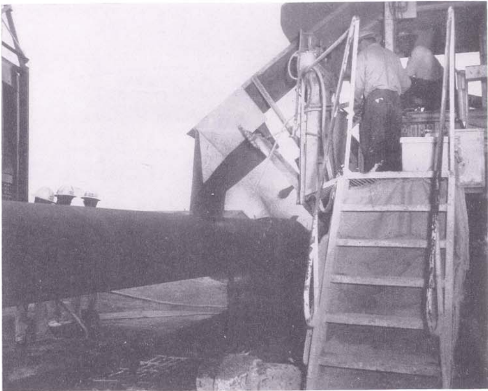
One of the pipe coating operations of H. C. Price Company on Peters Road on the Harvey Canal. This company puts protective coatings on pipe from 3 inches to 36 inches in diameter, including Hevi Cote (concrete), Somastic and Enameling. It also places interior coatings on pipe.
