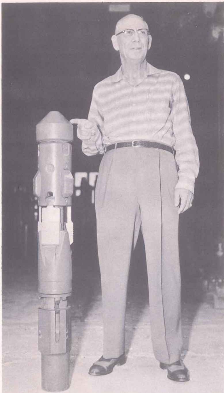
"This is a 7" cutter that can do its work more than two miles below the earth's crust," explains J. S. McKinstry, vice-president and general manager of Deltdel Fishing & Rental Tools, Inc., Located on the east side of Harvey Canal. "It is placed," continues Mr. McKinstry, "on the end of drill pipe and lowered into hole to desired depth. When in position it rotates and knives protrude and cut casing at desired spot. After casing is cut it is fished out of hole with a spear."
