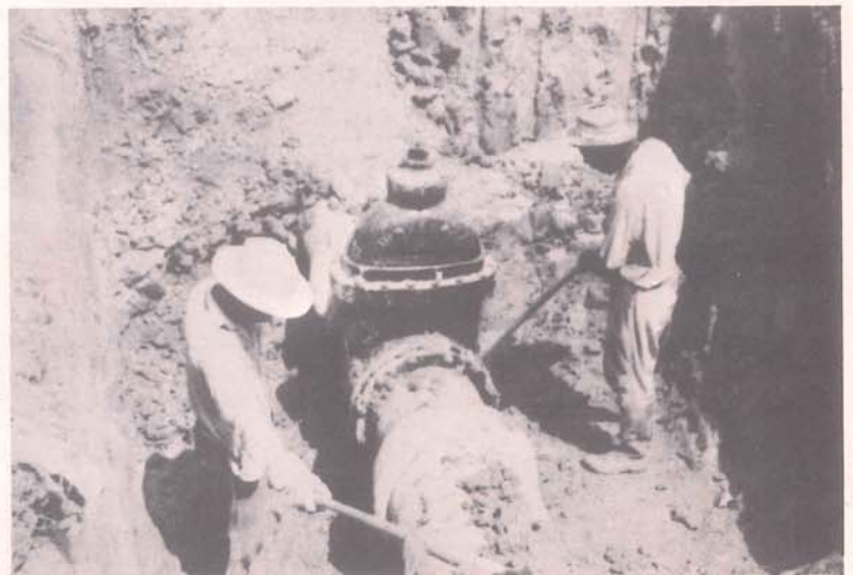
Two construction workers dig deep to install this 16 inch main valve which will control water pressure and feed the smaller pipe lines in Water District No. 3. The main valve is located on 16th Street between Avenue A and B.
