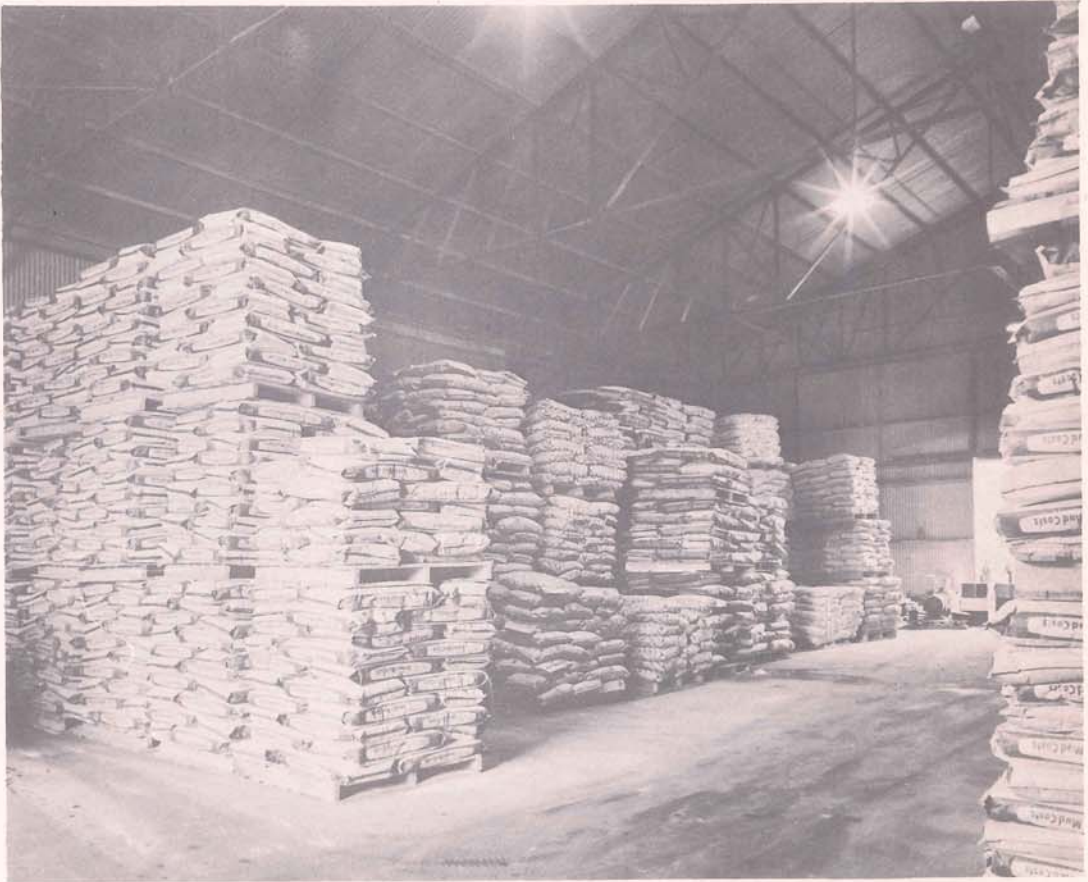
Bags of mud. Not the kind little girls use for pies, but drilling mud. Without mud there would not be any deep well drilling. Mixed with water and chemicals the solution is pumped into the hole to lubricate the bit; removes bit cuttings from the hole; seals walls; and prevents blowouts. Mayronne Drilling Mud & Chemical Company on the east side of Harvey Canal, where picture was taken, supplies this vital material to the oil and gas drillers.
