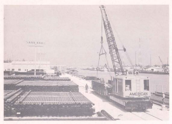
Shell Oil Company's marine warehouse and pipe yard on the Harvey Canal is equipped with a 25-ton diesel railroad crane for handling various sizes of pipe in the yard.
