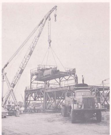
At left; loading a drawworks on offshore structure of Rowan Drilling Co., Inc., at Hunt Tool Company's yard on the east side of Harvey Canal. Below; stacks and stacks of lumber. In the background are some of the big timbers used for constructing tank batteries and bulkheads. The 12"x12"s on the yard of Harvey Lumber & Supply Company, Inc., on the east bank of Harvey Canal are creosoted Southern yellow pine.
