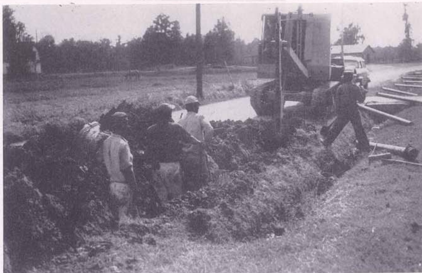
The mechanical digger nonchalantly chews out the ditch for a new water main on Manson Drive in Marrero.
