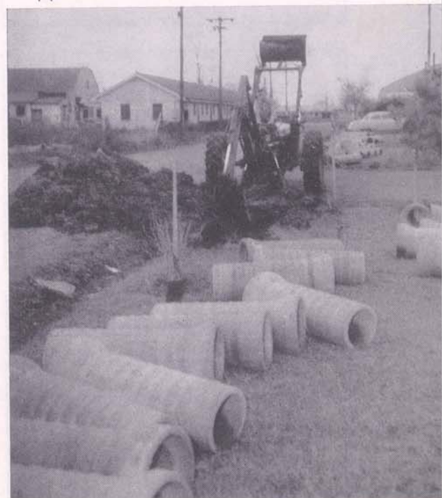
Digging trench to lay subsurface drainage pipe.
