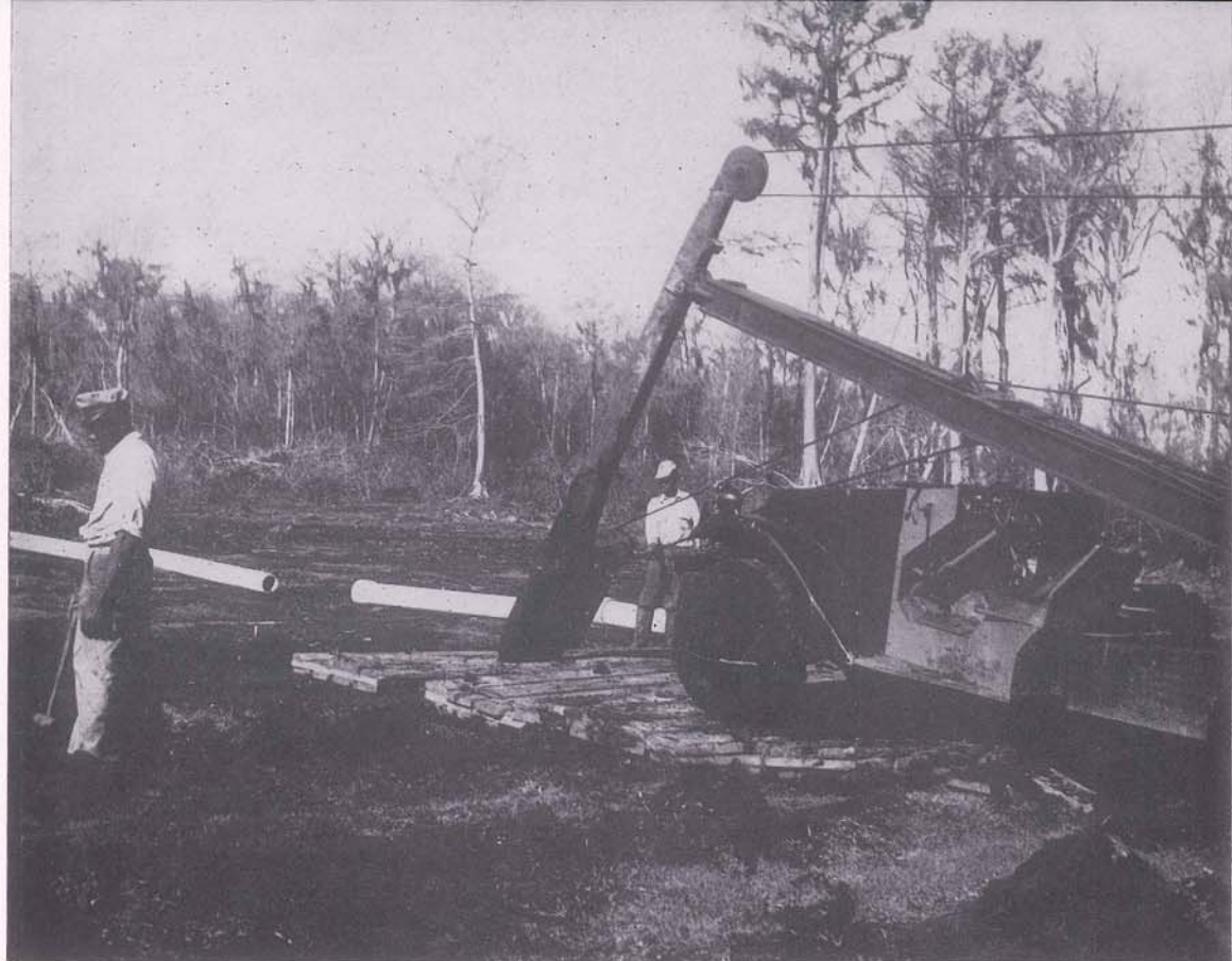
Laying water pipe in advance of construction on new Veterans Memorial Highway. Notice the clever machine that pushes its own road ahead of it.
