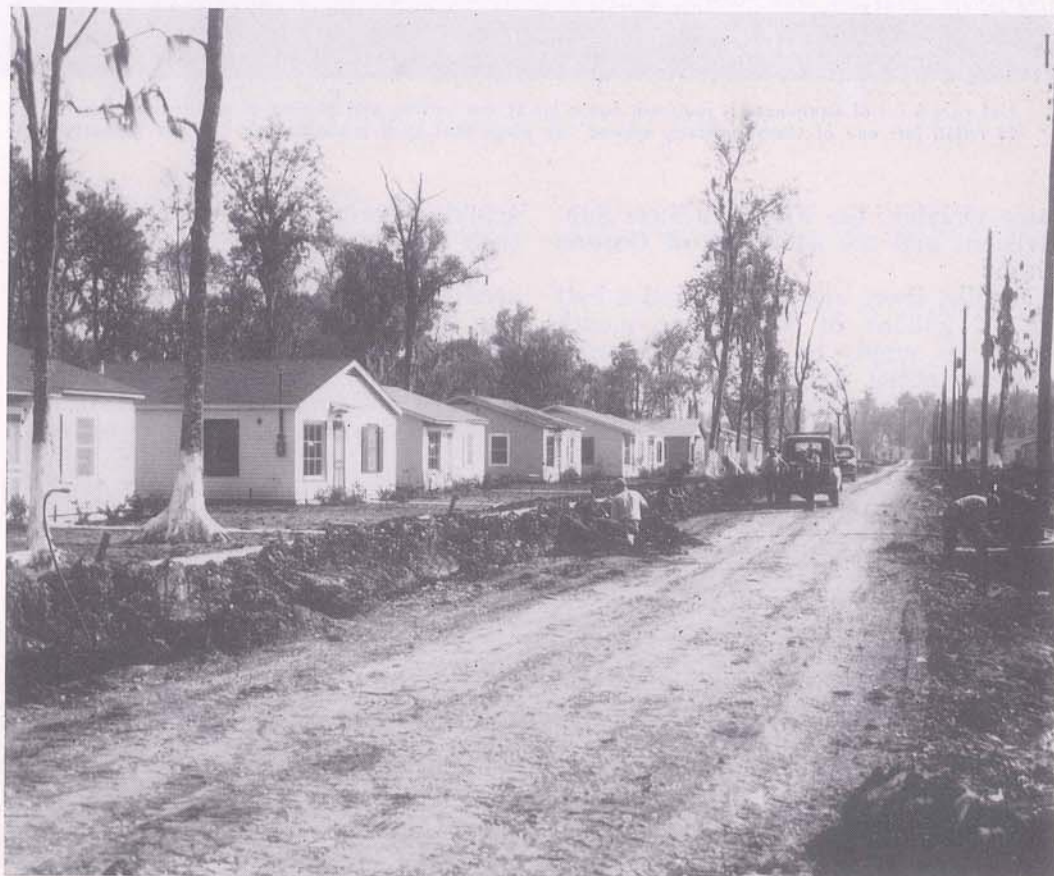
Showing "Operation Progress"—the laying of the water mains in a new Water District No. 3 subdivision, before the street paving begins.
