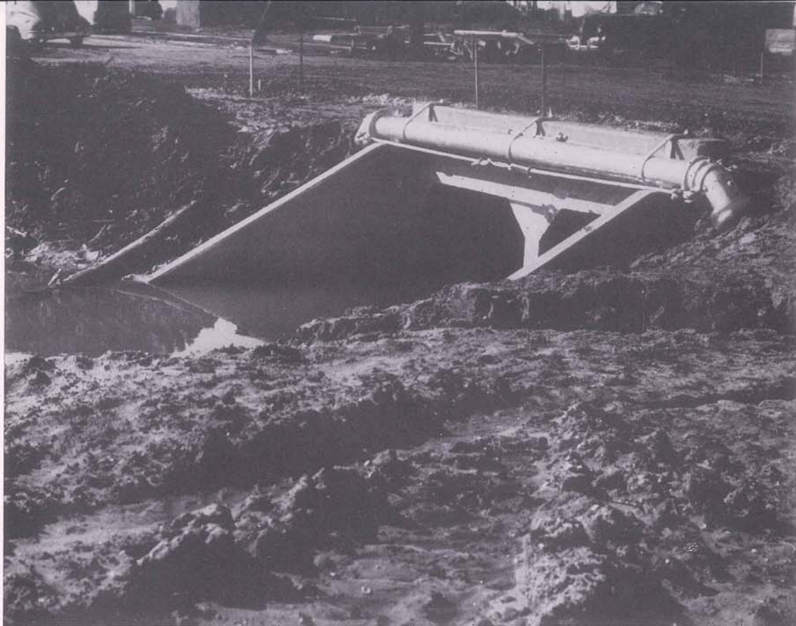
Showing method of running water pipe over a drainage canal before Veterans Memorial Highway was constructed.
