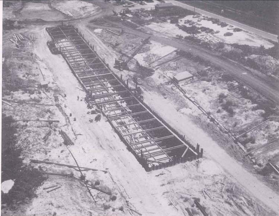
A 3-foot thick concrete slab, which forms the base for the roadway of the new Belle Chasse Tunnel under the Algiers cut-off canal, is housed in this steel coffer dam until the dam is removed for work on another section of slab. Through this new tunnel will be diverted Highway 31, from Venice to Gretna.
