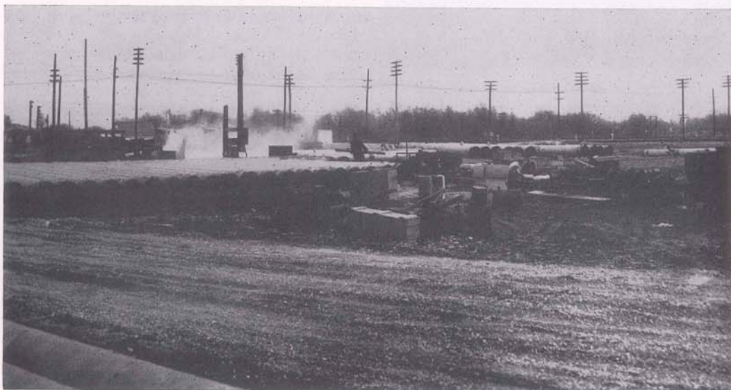
Coating and wrapping water mains by contractor before placing them underground.
