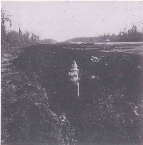
Installing the water main for one of East Jefferson's protective fire plugs on shoulder of new highway.
