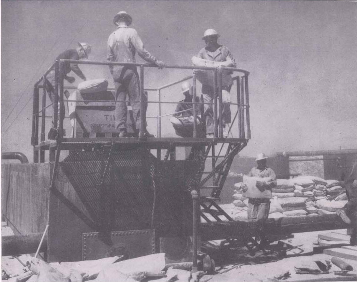
Mud, commonly referred to as "drilling fluid," is the life blood of an oil well being drilled. Shown here, through the courtesy of Humble Oil and Refining Company, are drilling crew members carrying sacks of the vital mud material to the mixing stand.
