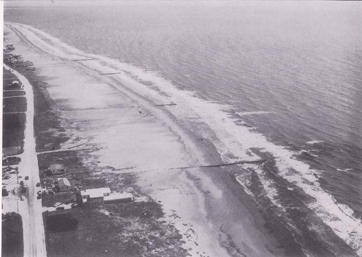
A segment of the famous eight mile long beach at Grand Isle, showing a few of the timber groins that have been constructed to recapture the precious sand lost by erosion. There are about sixteen of these groins altogether averaging around 500 feet long and spaced from 700 to 1000 feet apart.
