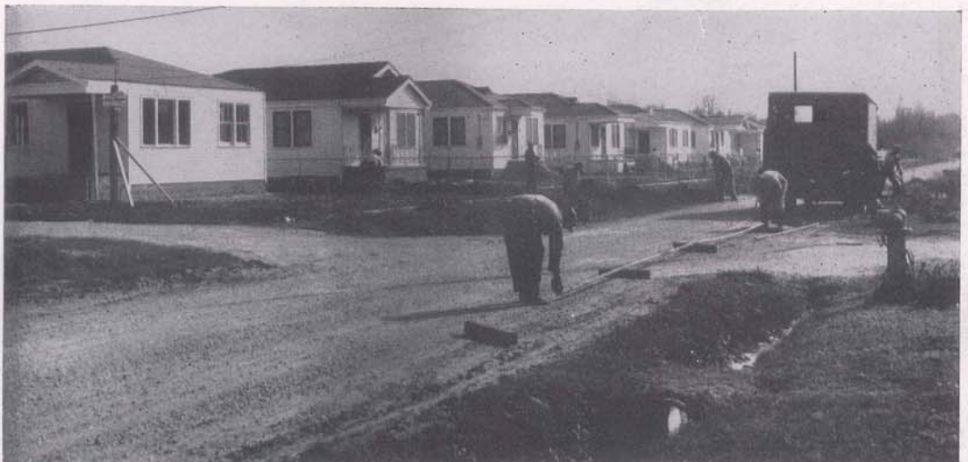
This is a Chipley Street view of Westwego's newest subdivision, showing a crew of the Louisiana Power and Light Company laying the gas mains.
