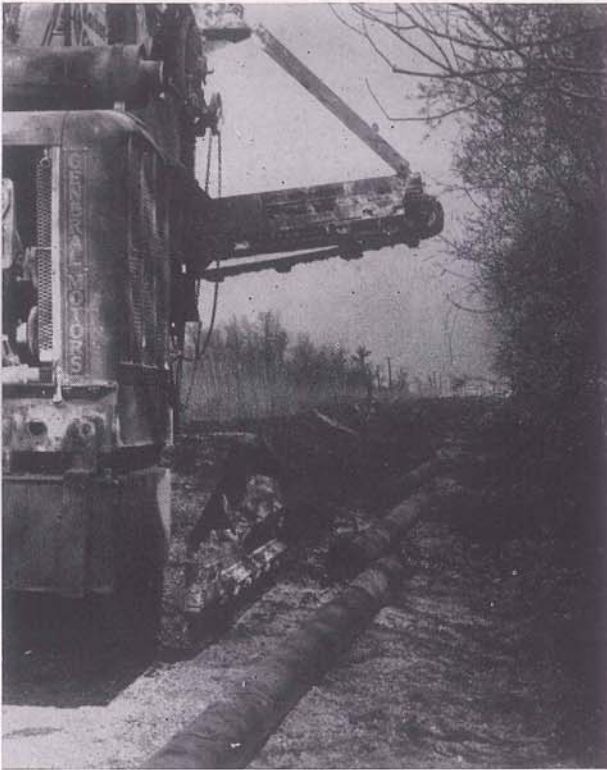
Part of the tremendous job of laying 8000 feet of 6 inch cast iron pipe along Peters Road on the East Side of Harvey Canal.
