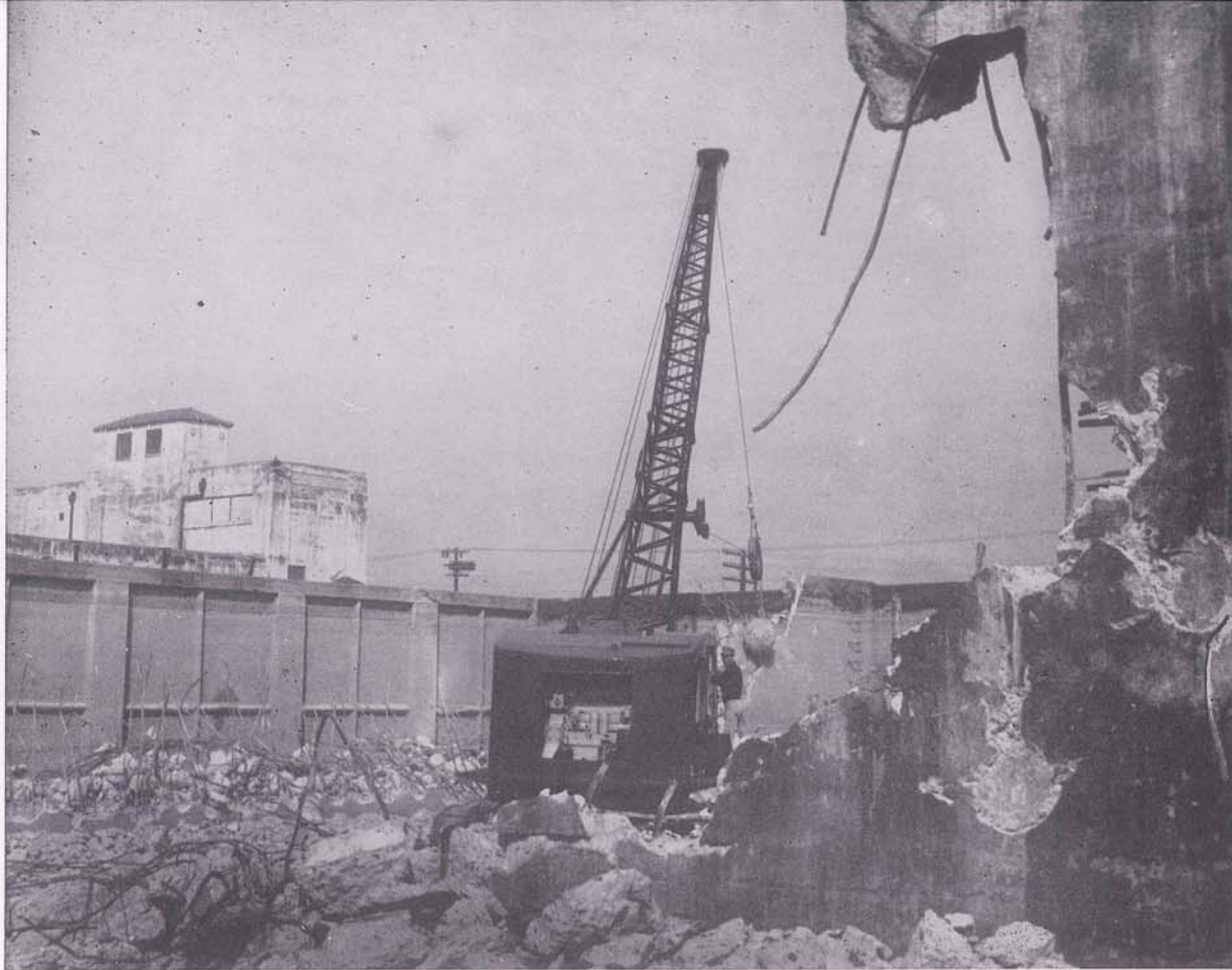
Progress at work at East Jefferson Waterworks District No. 1. . . . Here is shown the demolition of the old settling basins to make room for the building of part of the new plant.
