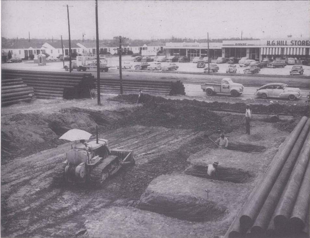
Excavating ground just off Jefferson Highway for a new treatment unit of East Jefferson Waterworks that will double the potential capacity of pure water from 10,000,000 gallons every 24 hours to 20,000,000 gallons.
