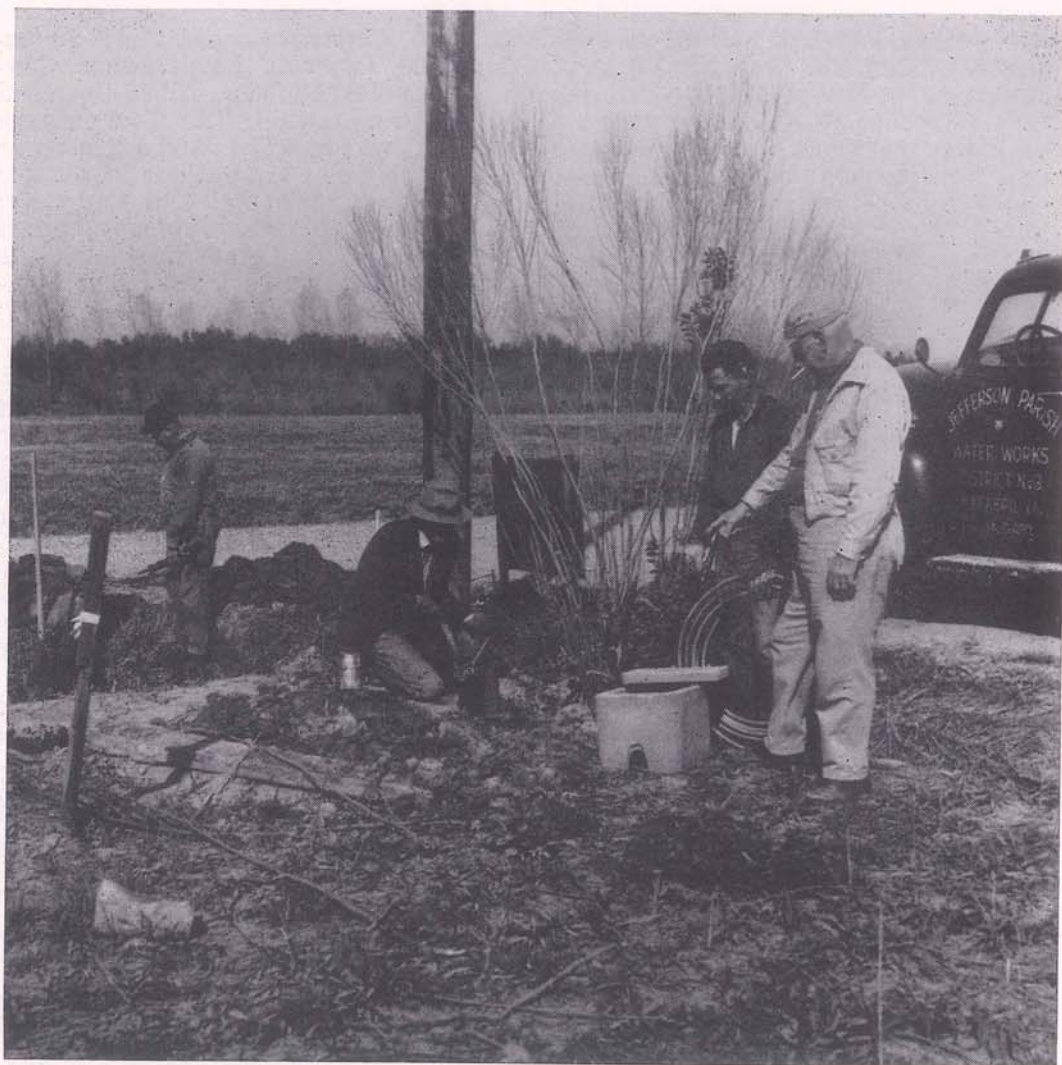
A crew of Jefferson Parish Waterworks District No. 3 installing a water meter with Superintendent O. A. Barnewold directing the operation.
