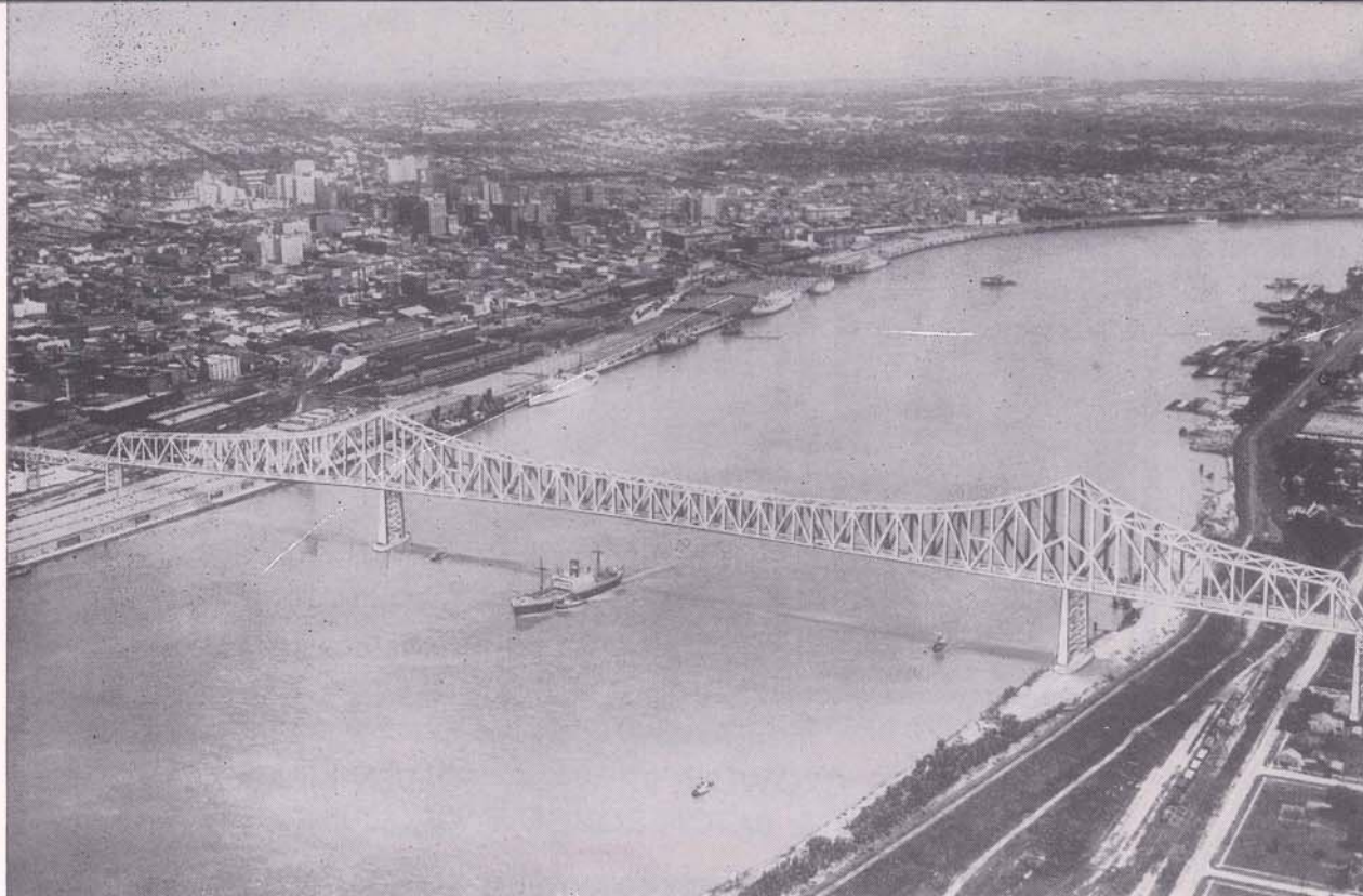
On Monday, March 16, 1954, the Army issued the permit for the erection of the Mississippi River Bridge as visualized by the above drawing prepared by Modjeski and Masters, Consulting Engineers. The plans call for the construction of a cantilever span 1575.33 feet long, with a 1400 foot long clear width for navigation, and a height 150 feet above high water. One of the piers will be in the river 555 feet from the East Bank. The Bridge will cost an estimated $54,081,000. The river is some 2000 feet wide at the proposed point of construction.
