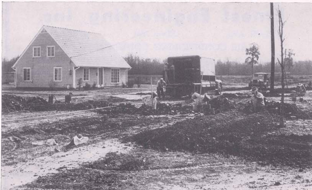
A picture of progress in Gretna—extending the gas main in the new Gretna Green Subdivision.
