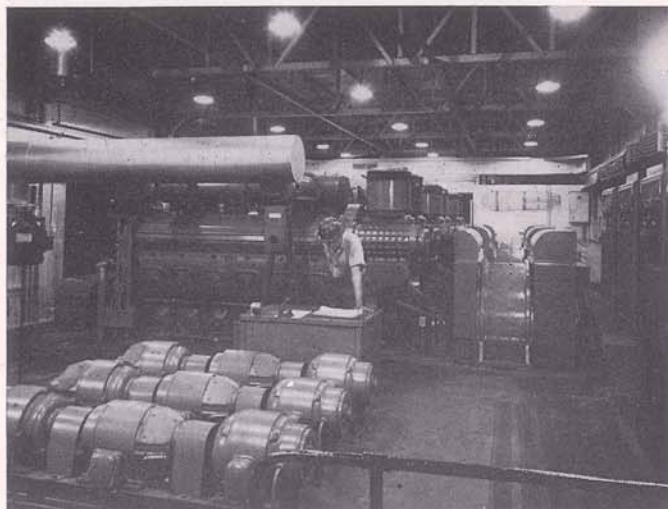
And inside this Humble Oil and Refining Company Power Barge are shown here the huge amplydine generators (see foreground) which regulate the power load from 3 thousand horsepower engines that drive the generators at right.
