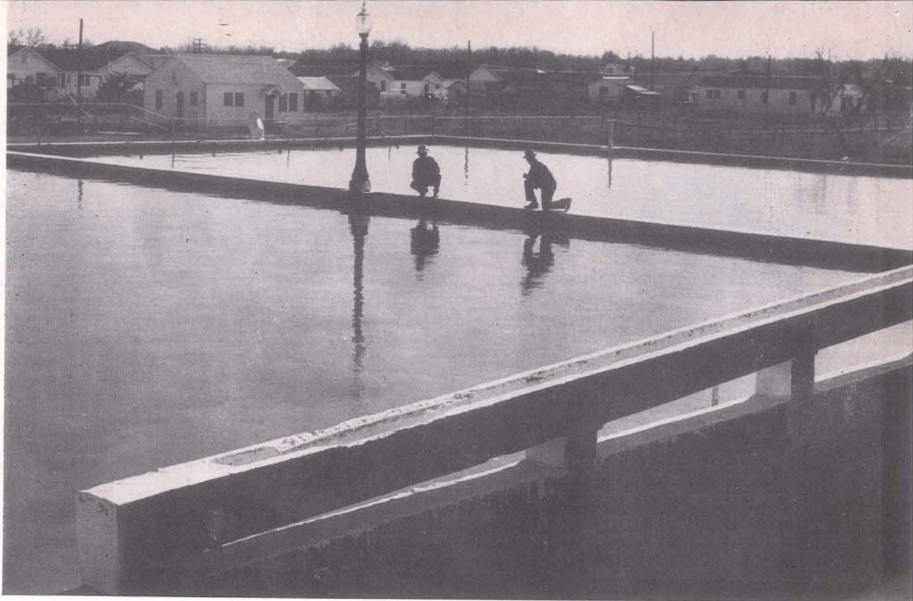
Settling basins of the Jefferson Parish Waterworks District No. 2, of 1,200,000 gallons capacity each.
