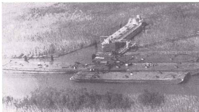
CRUDE PETROLEUM may be transported ashore, or stored in tank battery barge, as Gulf Refining Co.'s "Old Hickory", above. Oil is separated from gas on Gulf's oil production storage barge, below. At left is Texas Co.'s natural gasoline plant at Lafitte, La., where 12,000 gal. of the fuel are converted from natural gas daily.
