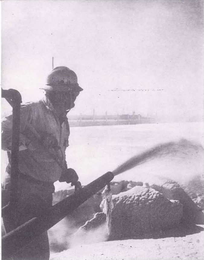
MOLTEN SULPHUR being sprayed on to storage or "vat" site at Freeport's Grande Ecaille mine in Plaquemines Parish, one of only two places in the nation where sulphur is profitably produced.
