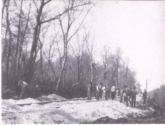
RAILROAD construction crew tamping ballast for tracks leading to new pipe covering plant.
