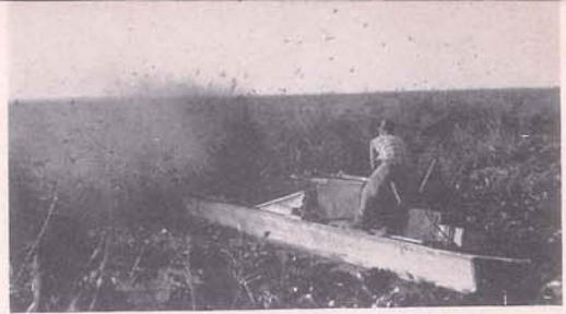
To dig canals back into Louisiana's trapping grounds, this unique but effective equipment is often used. Whirling knives on the front of this flatboat, driven by a gasoline motor, literally bore a waterway through the trembling prairie.
