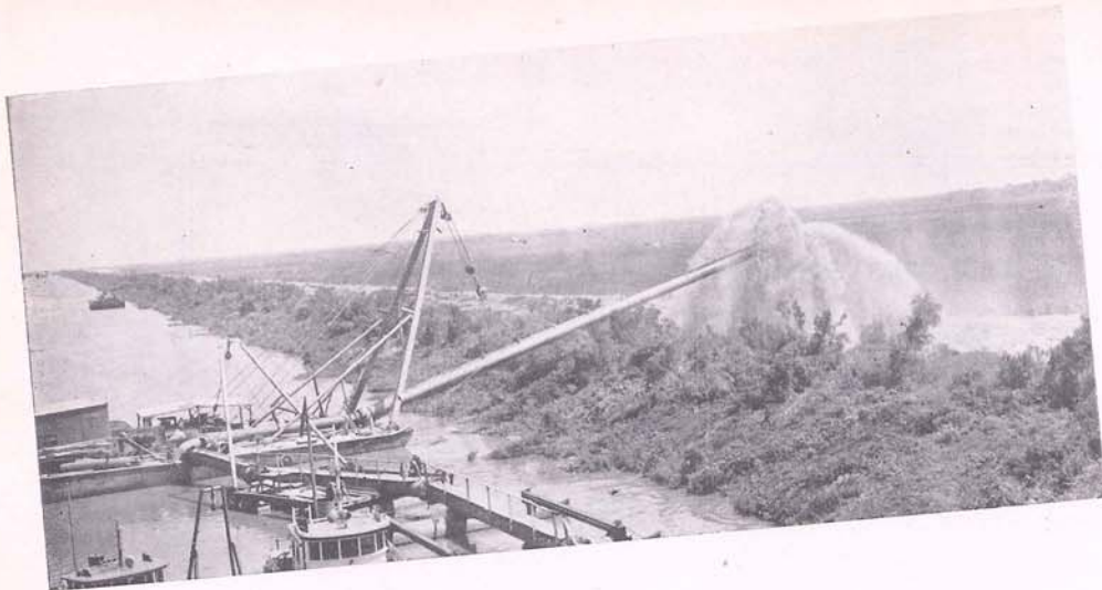
A Suction Dredge of this type was used recently to widen the Little Bayou Barataria link of the Intracoastal Canal. The photograph shows how the spoil is deposited beyond the Canal's bank.
