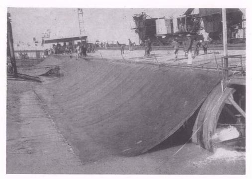
Corps of Engineers, U. S. Army, laying an asphalt mattress on the bottom of the Mississippi to prevent it from eating away the levee. Notice the gap in the mat for fitting the landward section around the Westwego Ferry landing pile structure. Men on top are stapling reinforcing wire preparatory to pouring the hot asphalt. About 200 men to a crew. Mats sometimes laid as deep as 90 feet.
