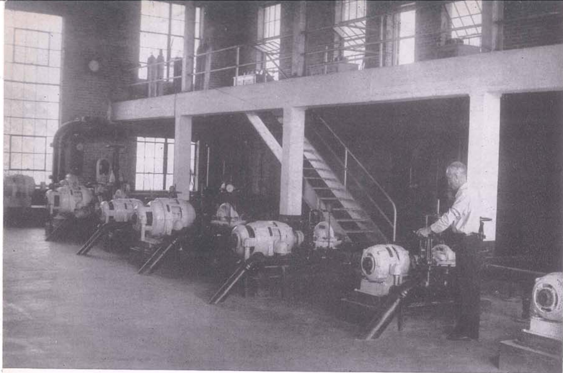
This battery of motors man the pumps at the Gretna waterworks.
