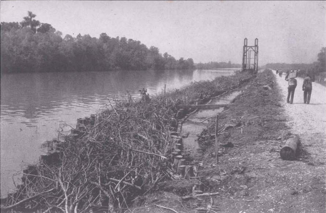
More than sixty-seven thousand hand-hewn cypress pilings will be driven in double rank on this canal project to hand-cuff Gulf tides and improve drainage.
