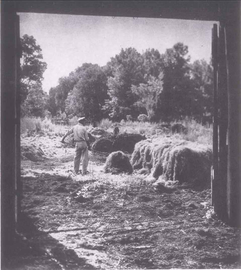
A man must fork his moss harvest after dampening it, in order to hasten the deterioration of its green vegetable sheath, yet prevent the rotting of the moss fiber inside. This fiber (black or rough moss) goes from picker to gin to market.
