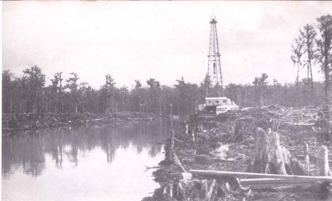
The California Co. drills from barges in the Barataria field. This canal was dug especially to give access to the proposed drill site, as water transport is more feasible than land travel through the marshes. The rig is on a barge, sunk in the canal to give a solid foundation for drilling operations.
