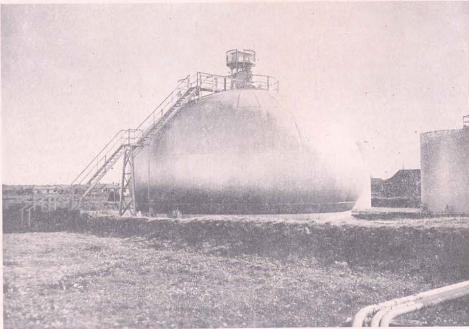
An oil storage tank on the Intracoastal Canal in Harvey. The odd shape of this tank allows more volume.
